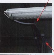
The view of the light inside the work area. Conduit screws into back of the box and hangs from the tube
