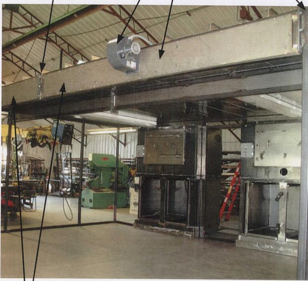
Bolt the left and right front header are to bolted together on the floor and lifted in place by a forklift. If your front is three piece you will have left and right POSI Air and the other is the center. Tighten the center bolts up before lifting in place. Locate all the bolts on the ends before tightening any of them.
